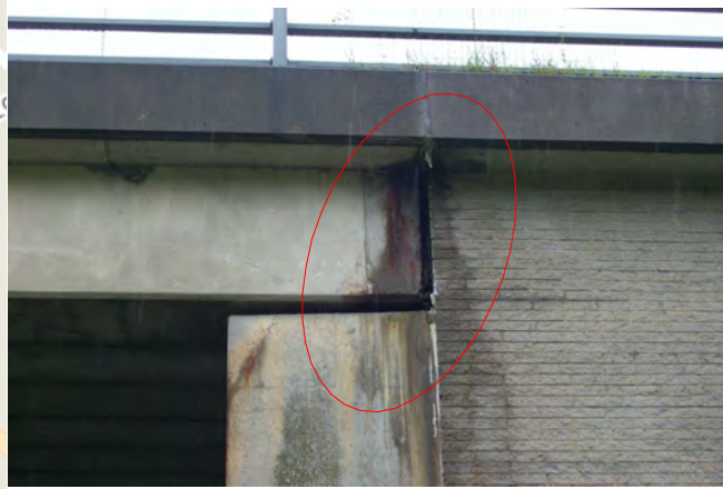
Photograph 1+2 North Elevation - Staining at bearing level
