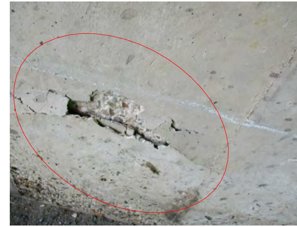
Photograph 1 , 2 and 3 Typical view of spalling of concrete at abutment wall
