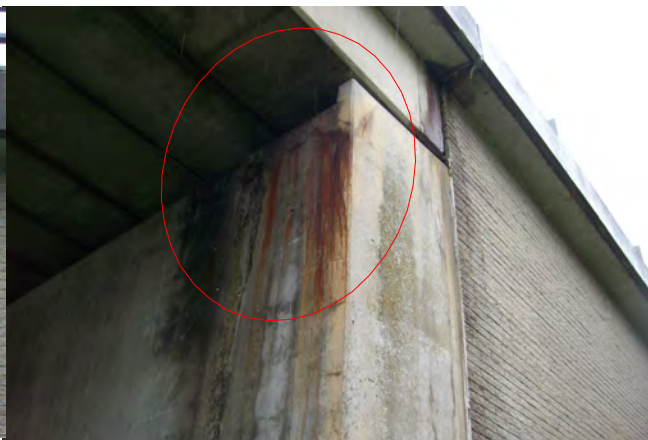
Photograph 1+2 North Elevation - Staining at bearing level
